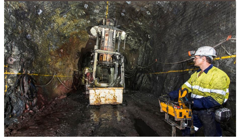
Rock bolting, Lady Loretta mine
