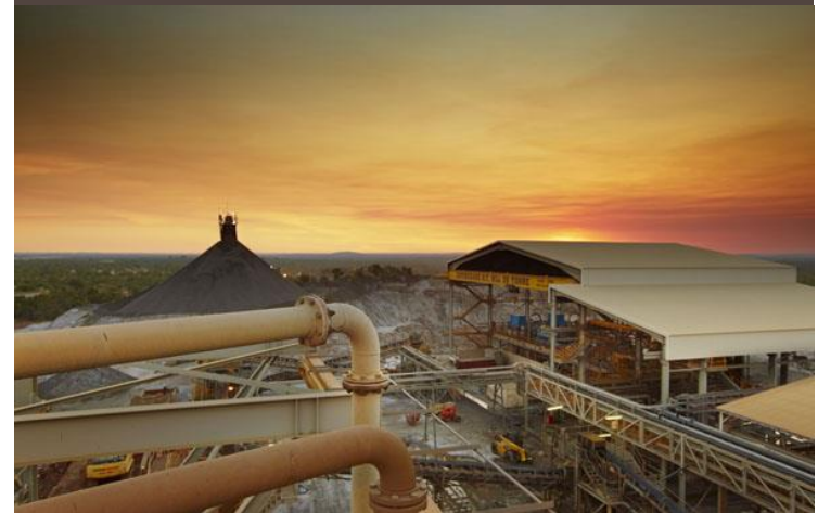
MRM Processing Plant
